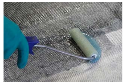
Wet lay-up with SikaBiresin CR168
